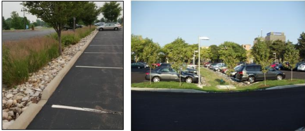
Figure 3.311-3: A combination of interrupted curbs (left), curbs, and wheel stops (right) can effectively allow flow of storm water into interior islands.
